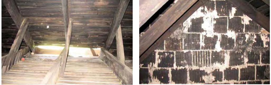
*Figs. 16 left; and 17, right. Views in the roof truss area, West Wing. Left: damaged and missing sheathing, north side of west wing, near end wall. Right: clay tile gable end wall.*
