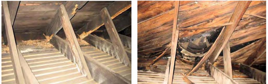
*Figs. 18 left; and 19, right. Views in the roof truss area, East Wing. Left: termite damage at north side; extent extends approximately five bays. Right: water damage to sheathing, and missing sheathing, south side.*
