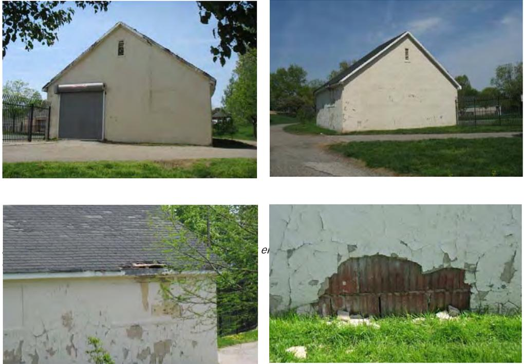
*Figs. 9, left; and 10, right: Left: Detail at wall and roof of East wing, south side, showing plaster condition and damage to roof sheathing near gutter (missing). Right: West wing, north elevation, showing an area where the stucco is delaminating and actually missing from the back-up clay tile wall system.*
