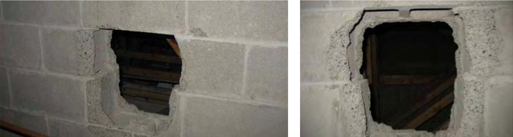
Figs. 12, left; and 13, right. Views in the roof truss area. Left: unprotected access hole through fire wall on west side. Right: unprotected access hole through fire wall on east side.
