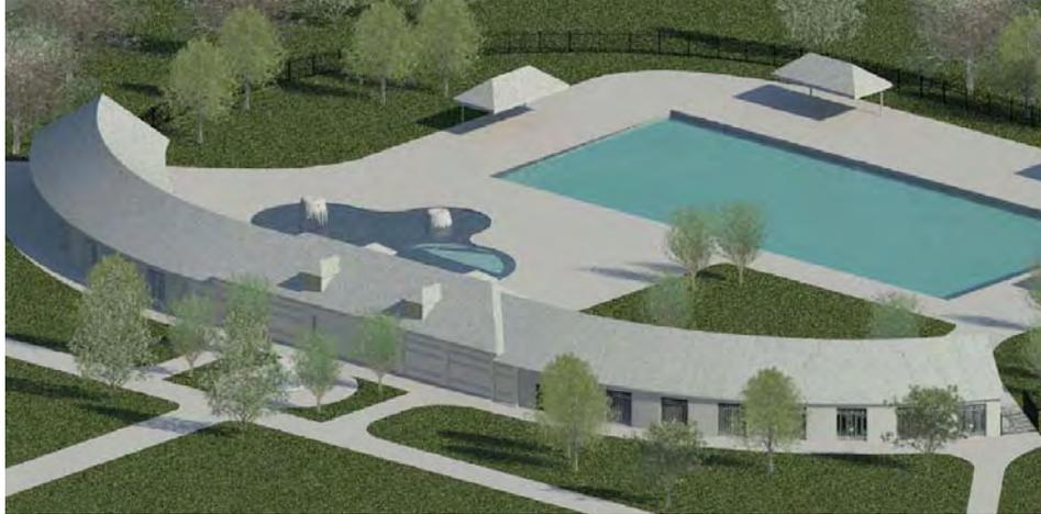
*Image 9 – Northwest bird's-eye view of Option 2. Walls at existing window locations have been removed and openings are gated at park side.*
