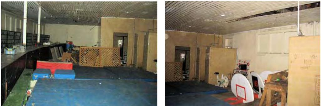
*Figs. 22 left; and 23, right. Views in the first floor area, East Wing. Left: general view looking toward southeast end wall. Right: general view looking toward south wall. Several areas of ceiling slats require work.*
